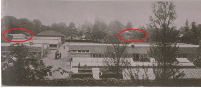
Figure 4.5 A centre of circulation: the iron room at Kew (highlighted left), showing its proximity to Museum No. 2 (highlighted right), c.1920s. © Board of Trustees of the Royal Botanic Gardens, Kew.
